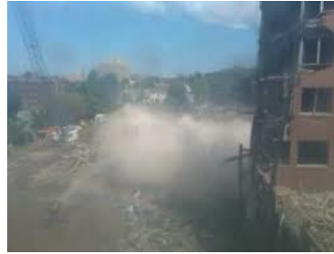
demolition of Genesee Hospital
